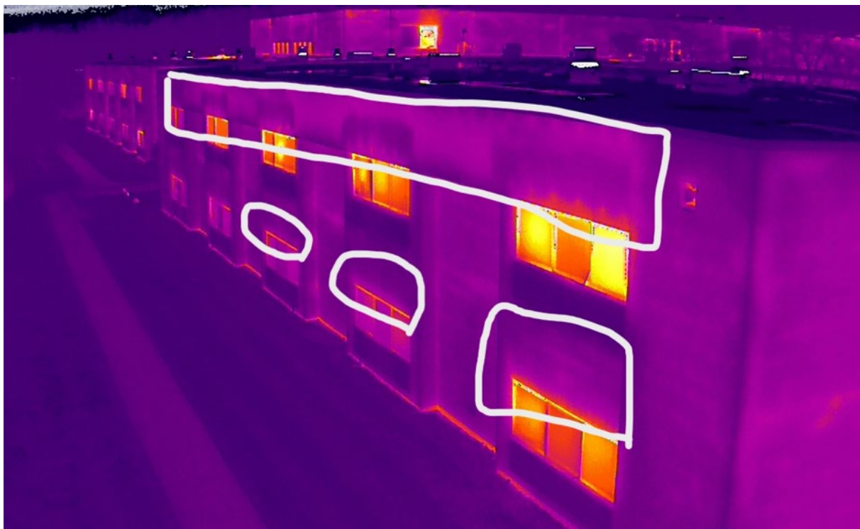
Image 2.17: Northwest Classroom Elevation Thermal Scan
