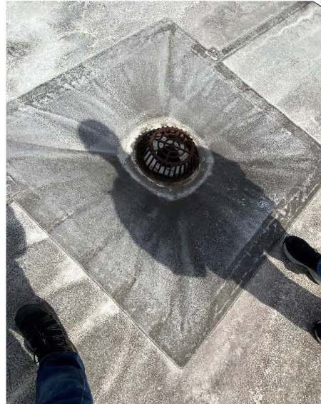
Photo # 24: Roof drain.
