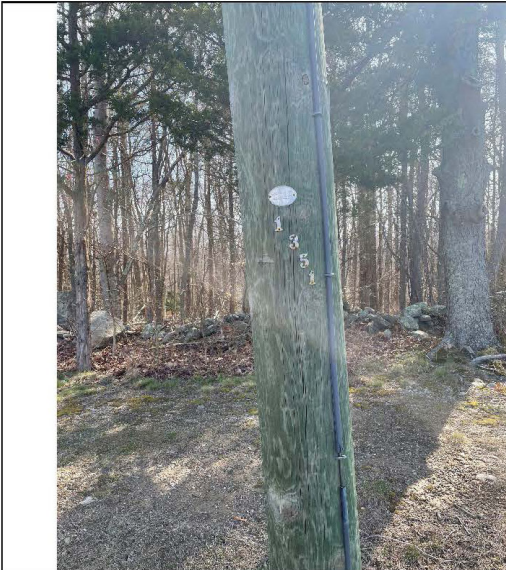
Photo # 25: - Utility Service Pole #1351
