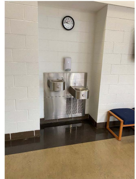
Photo # 2: Existing drinking fountain.
